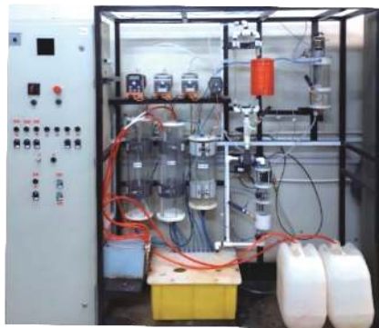
Fig. 6 Neutralization pH process plant
